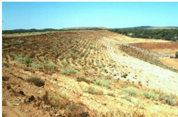
Figure 2. On a mine, a constructed slope has been contour ripped to produce a “bank and trough” system aimed to regulate resources. There are no signs of lateral flow in the troughs and hence no rills or gullies have formed on this slope.
